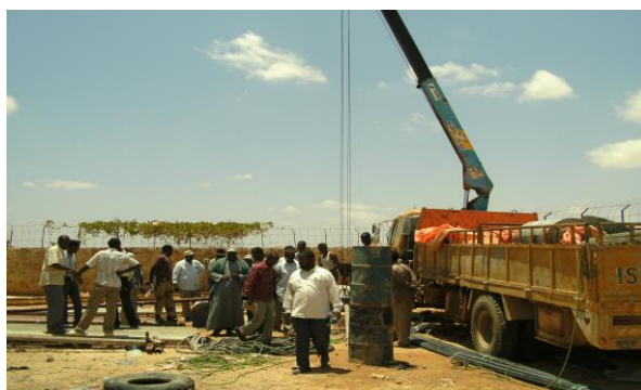
Rehabilitation of water wells
