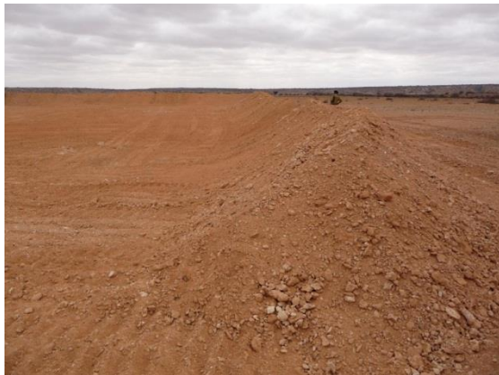
Plate 13 The recently constructed solid waste dump outside Gardho, which is awaiting the digging of drainage to prevent the site from flooding during the rainy season. Local authority staff highlighted that the site had yet to be formally handed over.
