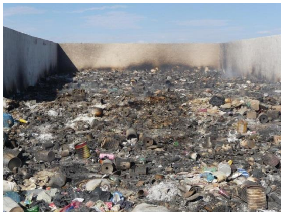
Plate 32 Recently constructed waste transfer station. The contents of the site were burned during the night by an arsonist. Storing solid waste in large quantities in waste transfer stations poses a direct fire risk to local residents.
