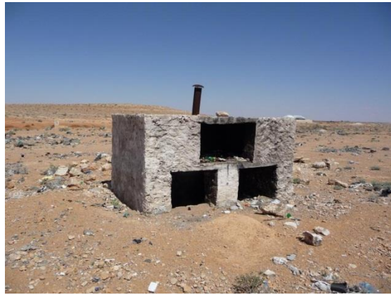
Plate 10 Locating the incinerators in an open public area with no restrictions on public access reduces the infection control measure of the facility if it was indeed working in the first place.
